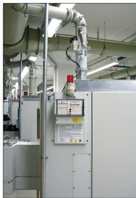
Control system for automatic fire system in conjunction with mist extraction protection
