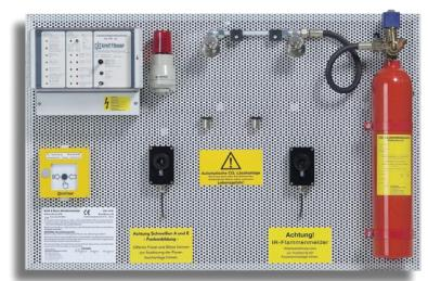
The corresponding fire detector releases a signal to the extinguishing system control
